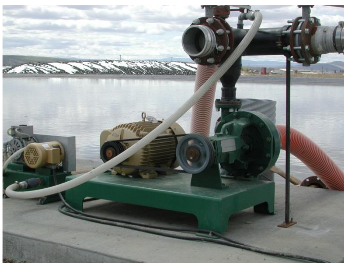
New electric pump for waste transfer after switching from an old diesel-powered PTO pump
